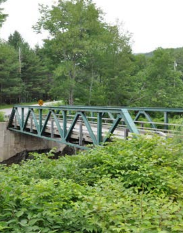
Lover’s Lane Bridge (below) is a rare example of a Warren pony truss bridge. It was built in 1918 spanning the Dog River and joining Chandler Road to Route 12.
