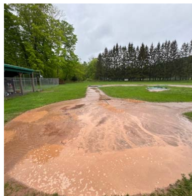
Photo 2: Rain runs down the basepaths and pools around home plate. Lack of re-grading means water ponds in the dirt and turns to mud.
