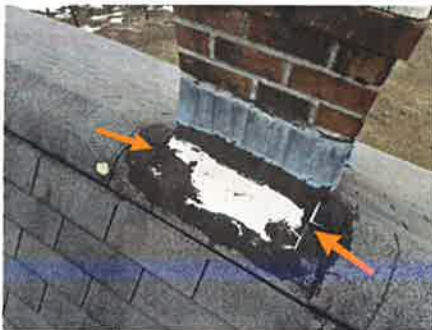
Poor repair
