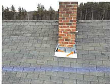
Loose counter-flashing
