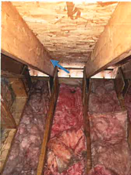
Soffit vent with no proper-vent channel
