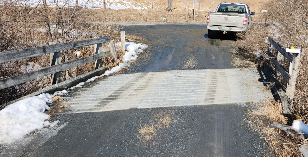
Top of Bridge, looking Northwest
