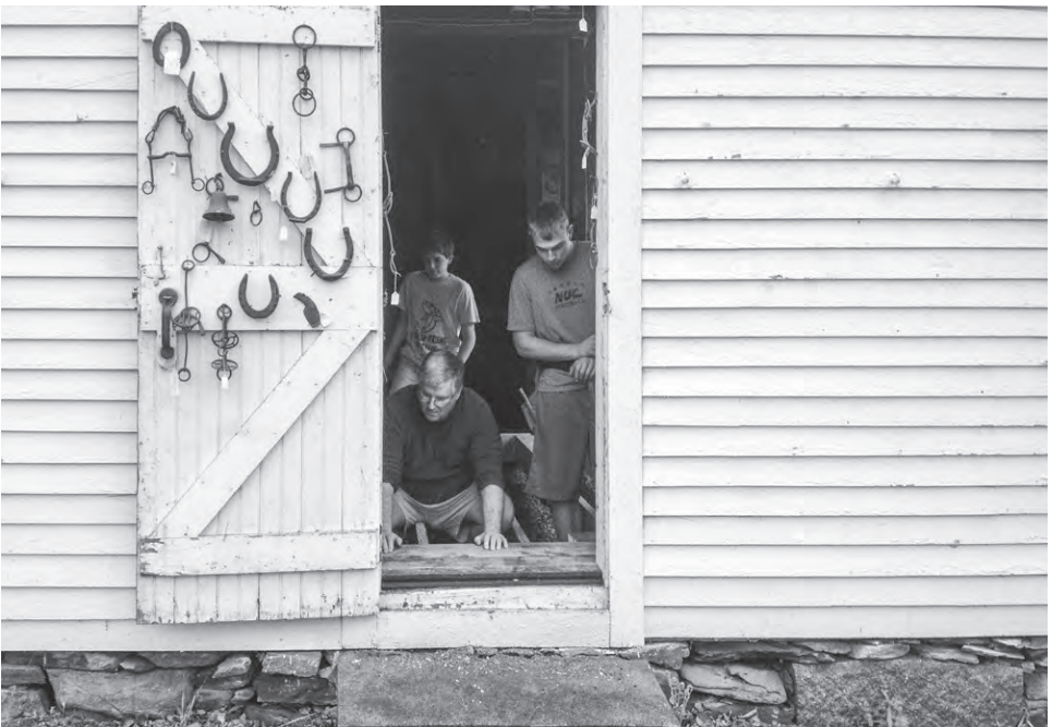
Norwich Scouts led by Joe Porter build a new floor for the Historical Society's tool shed as a community service project.
