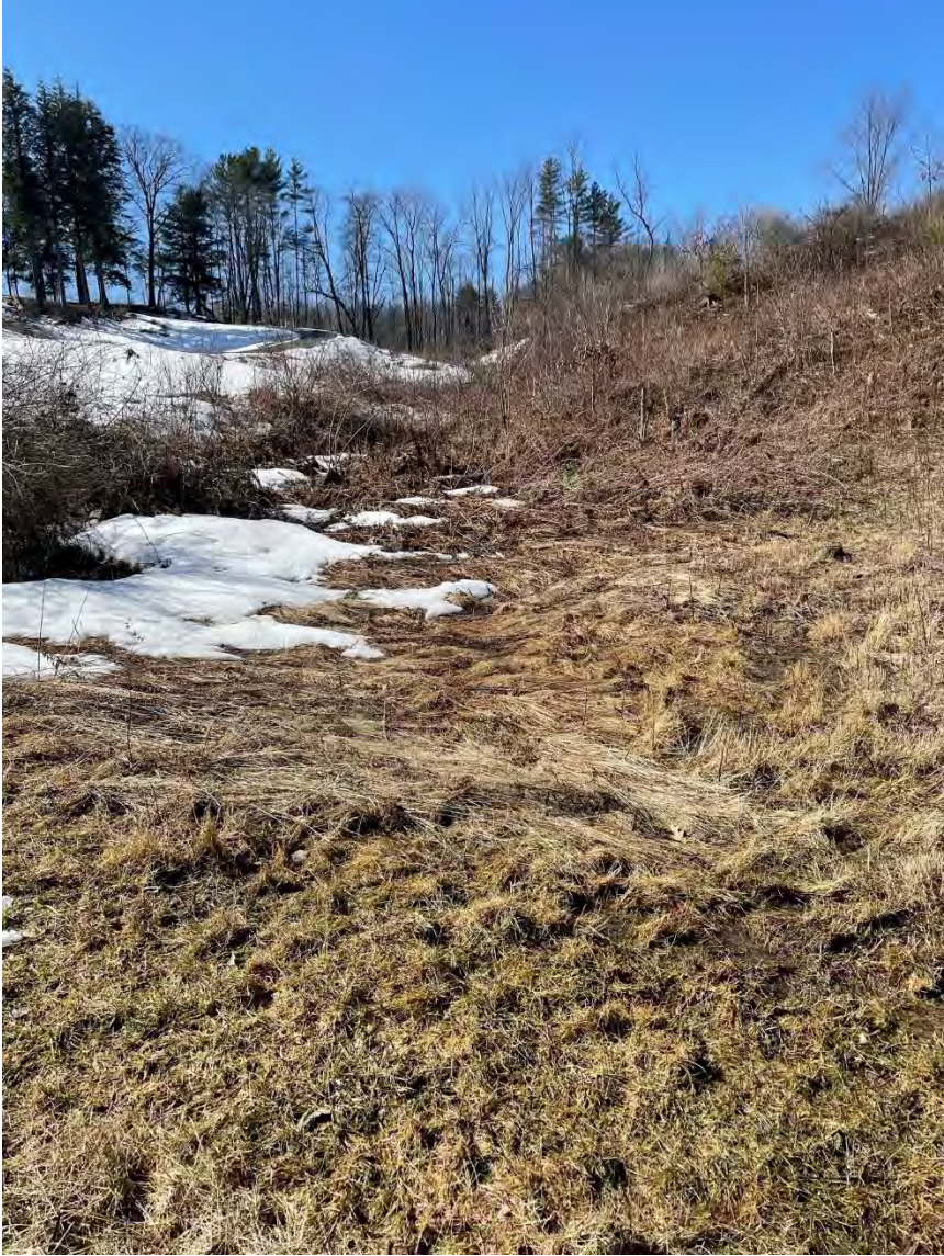
Looking upstream channel from culvert inlet
