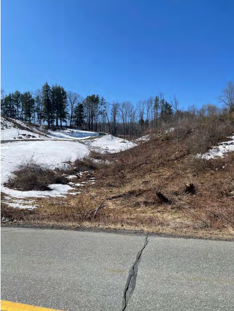
Looking upstream towards culvert inlet
