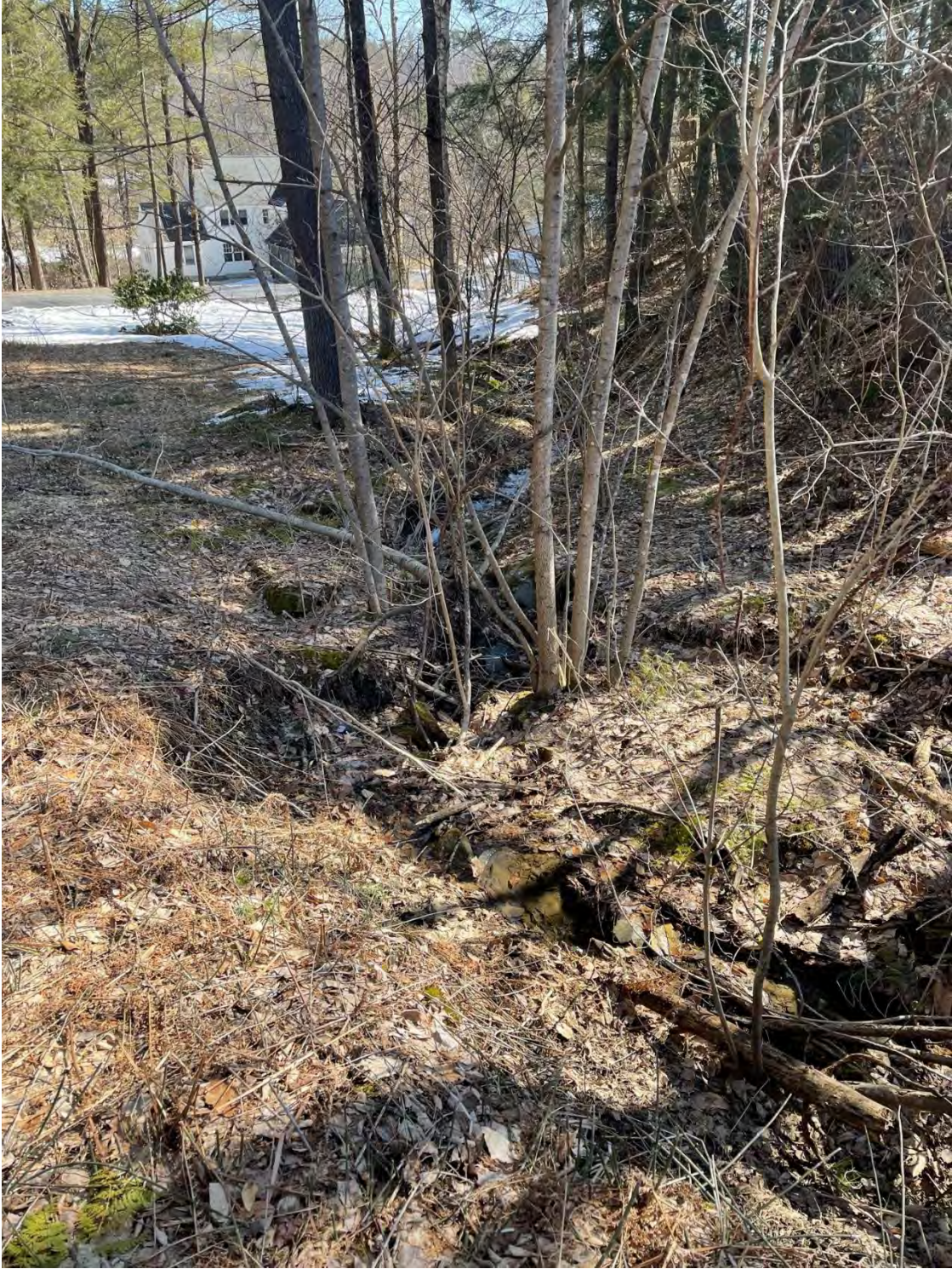
View of culvert outlet from VT132 roadway
