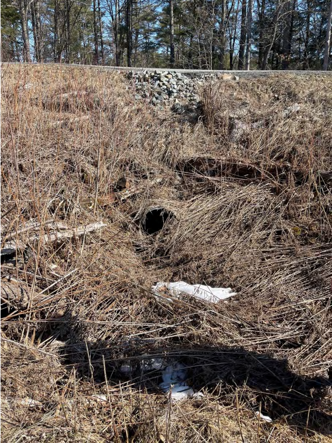
Culvert inlet view
