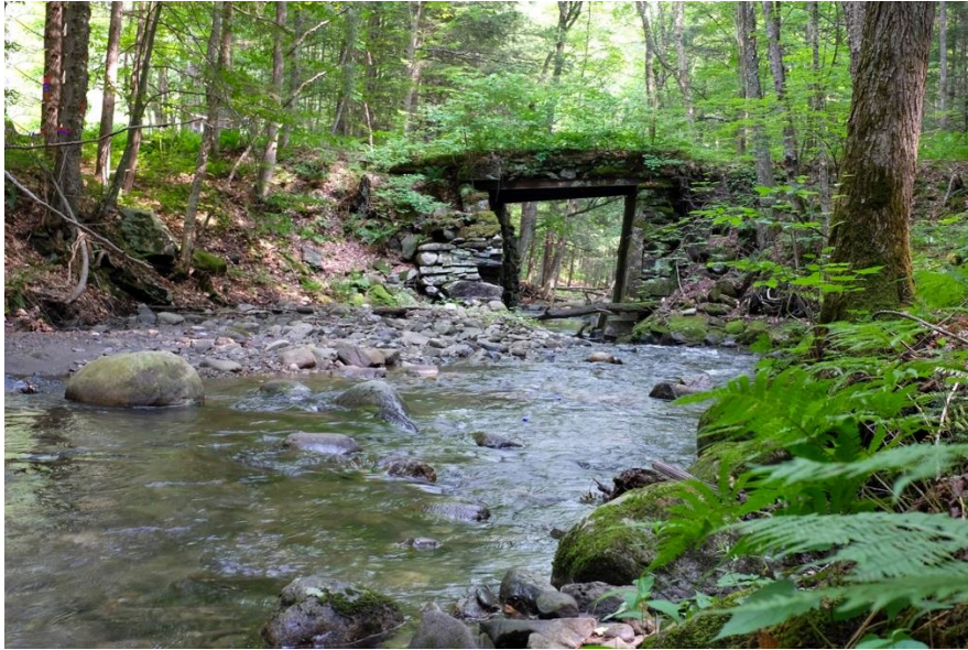
Bridge over Charles Brown Brook before 2018 collapse (Photo: P. French)
