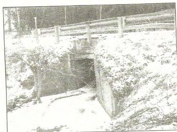
Figure 3: Poor condition box culvert
