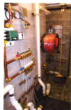
IN-FLOOR RADIANT HEATING
