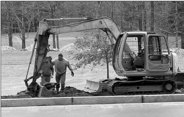
Installing sidewalks at Huntley Meadow. Photo courtesy of The Norwich Times.
