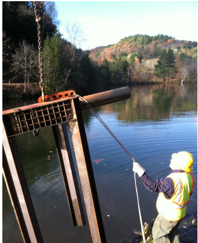
Sonny Lewellyn from Norwich DPW "steers" the Old Bridge dry hydrant into position as Graham Webster lowers it into the river. Photo by Steve Leinoff
