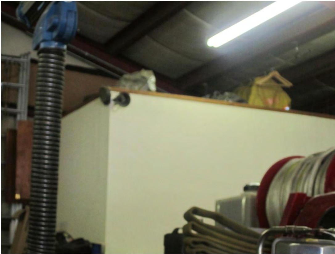
Photograph No. 12: Exhaust extraction hose system and open storage beyond.
