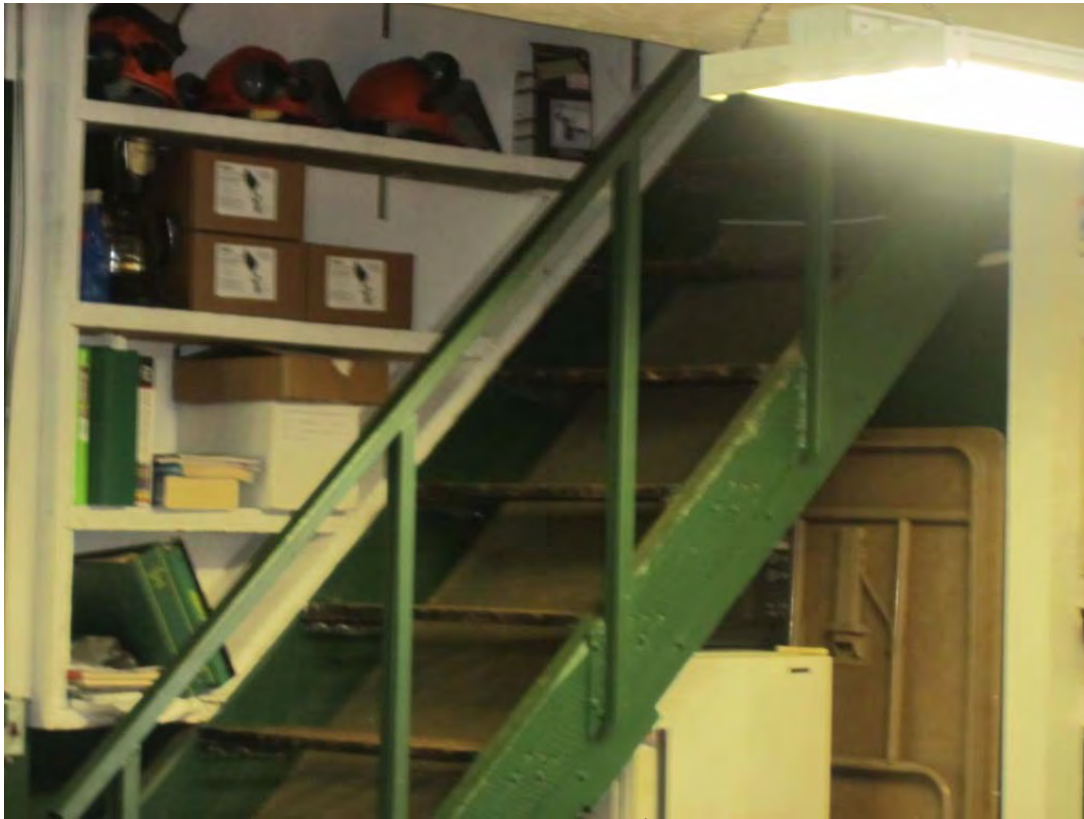
Photograph No. 5: More of the stairway to the 2 nd level that needs mid-rail.
