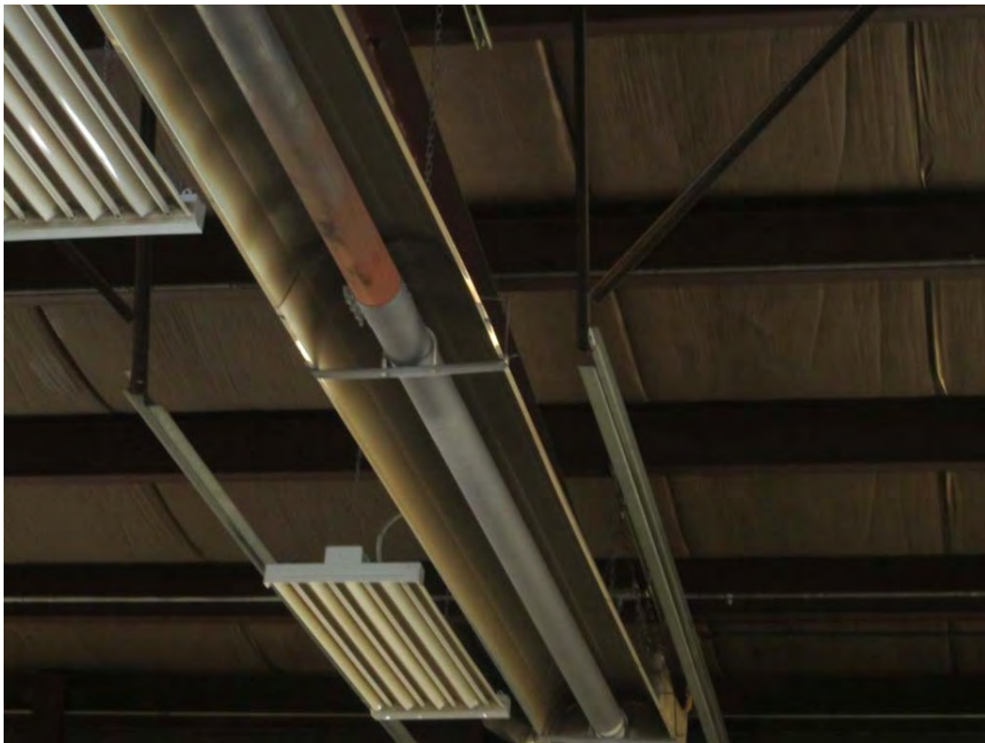
Photograph No. 10: Heat piping for convection style heat system.
