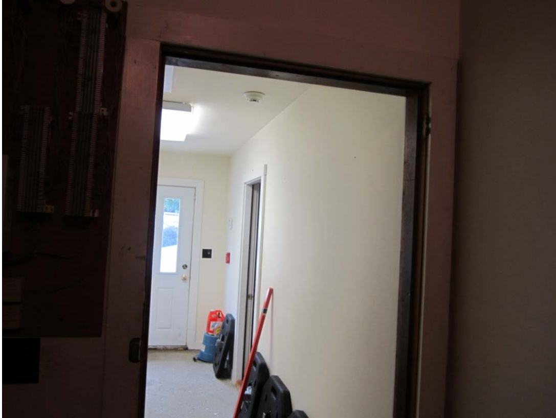
Photograph No. 1: Exit hallway to garage entrance.
