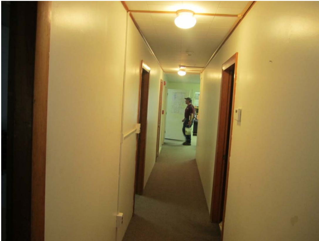
Photograph No. 5: Narrow corridor from Fire Chief office looking toward conference room and front entrance.
