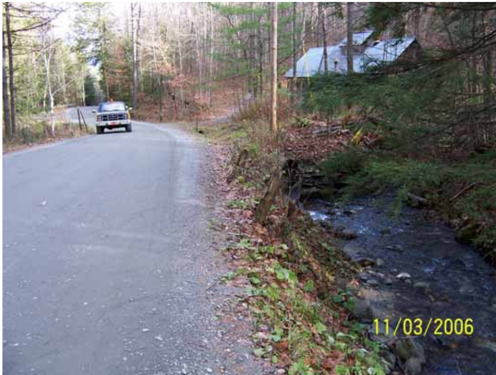
Bragg Hill Road Culvert Inlet
