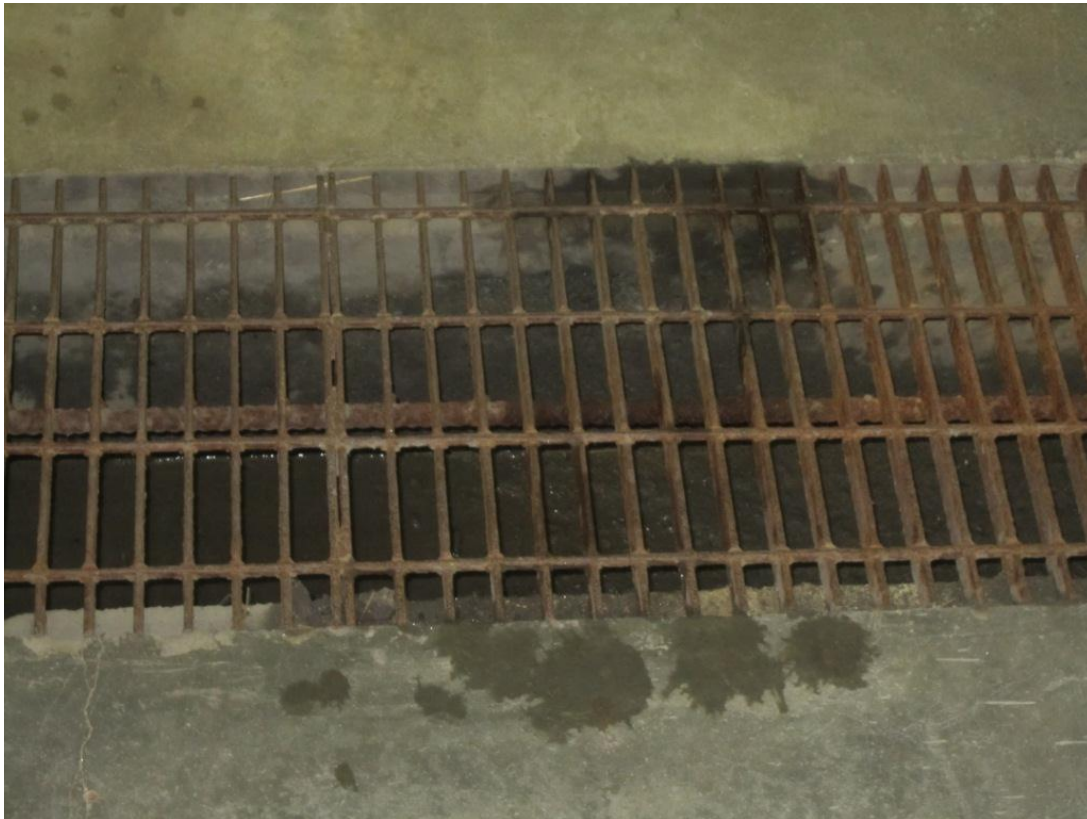
Photograph No. 11: Open floor grate that runs full length of the building.
