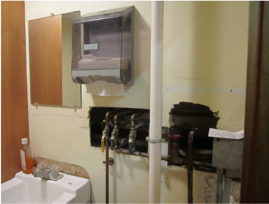
Photograph No. 4: Bathroom with holes through the wall into furnace room.
