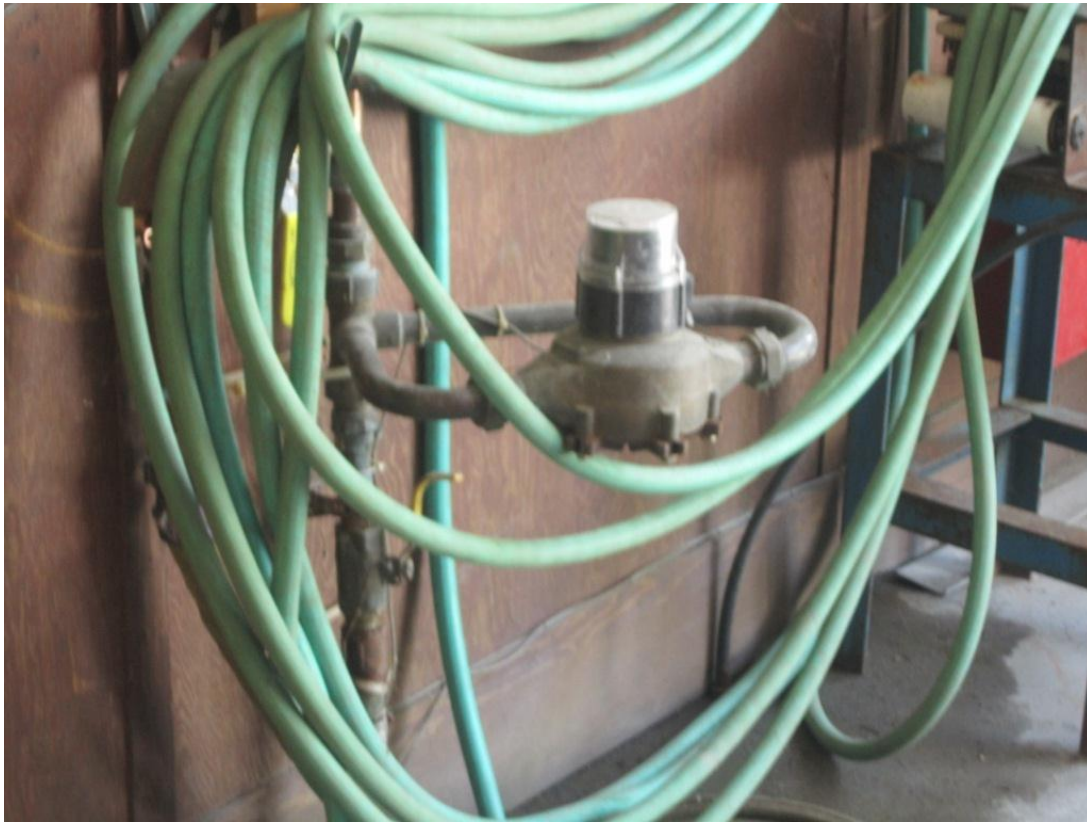
Photograph No. 14: Town water meter without backflow prevention.
