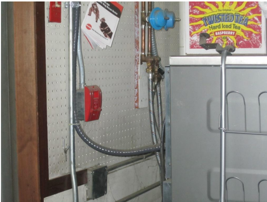
Photograph No. 7: Washing machine with partially hidden pull station.
