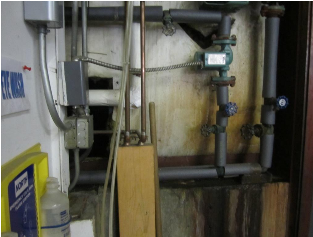
Photograph No. 6: Holes in the wall through to the furnace room from outside the bathroom and from the main Fire Station building.
