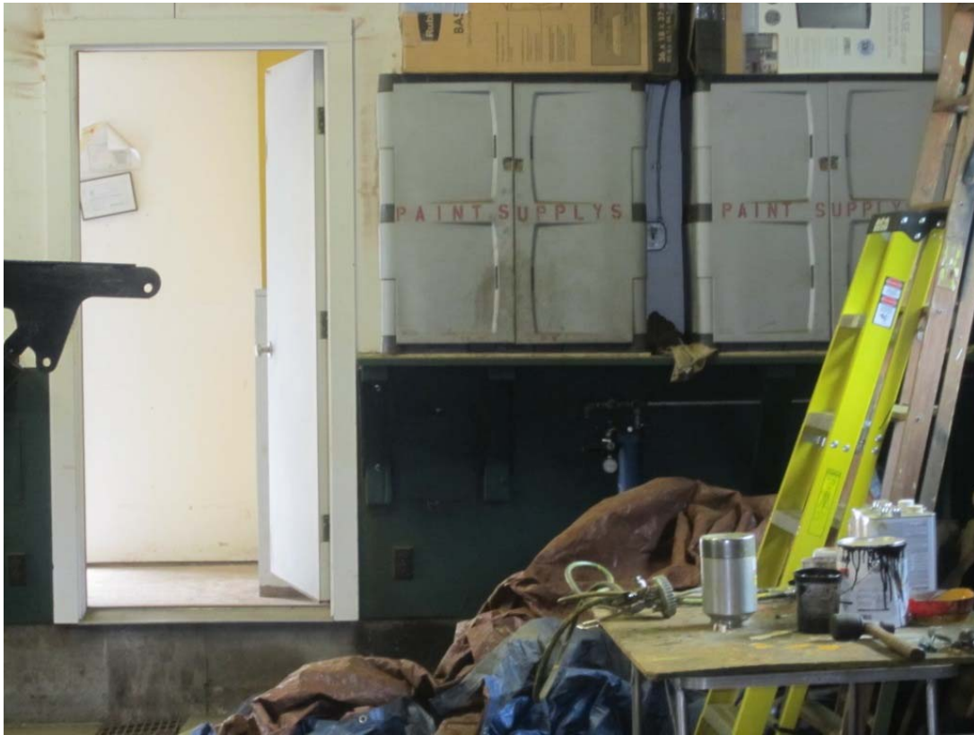
Photograph No. 9: More Flammable cabinets and oversized step up into generator room.
