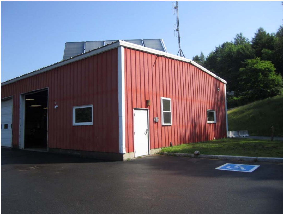
Photograph No. 17: Exterior of the existing building with solar panels.
