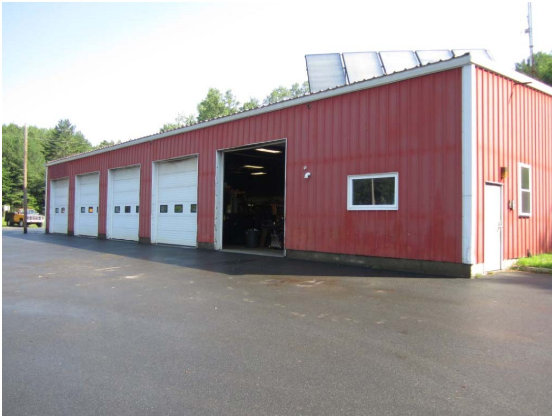
Photograph No. 16: Exterior of the existing building with solar panels.
