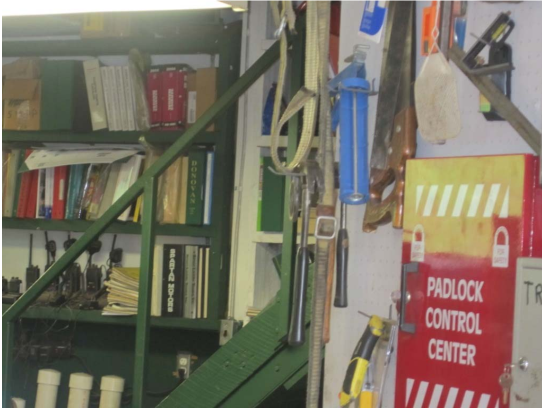
Photograph No. 1: Stairway going to 2 nd level of DPW that needs mid-rail at the least.
