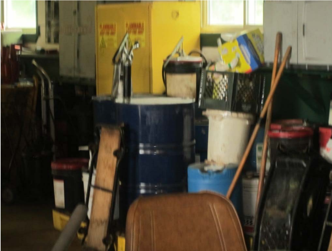
Photograph No. 3: More flammable fuel oil storage in bulk in the main DPW maintenance shop.
