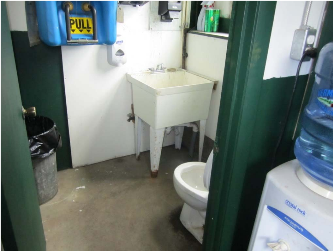
Photograph No. 14: Existing bathroom and eyewash station.
