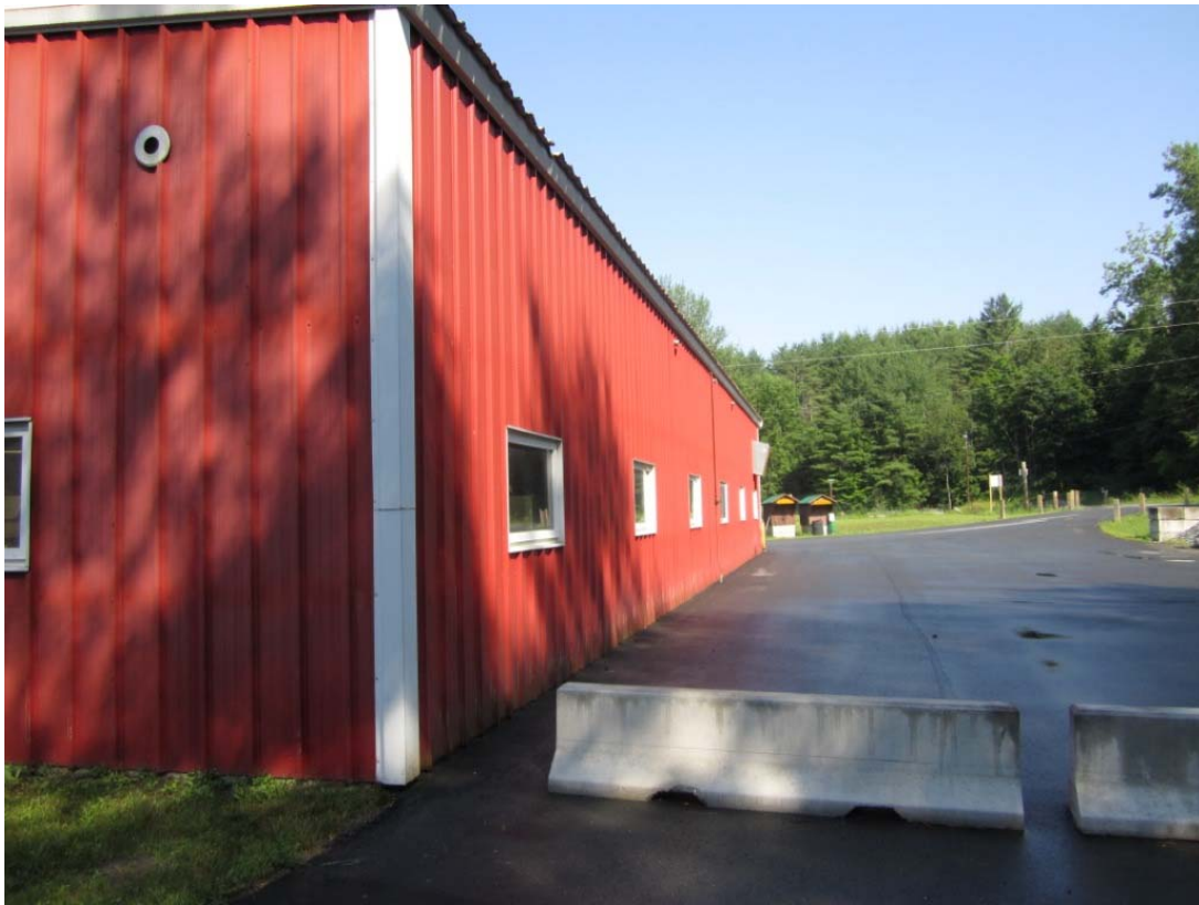
Photograph No. 18: Exterior of the existing building with solar panels.
