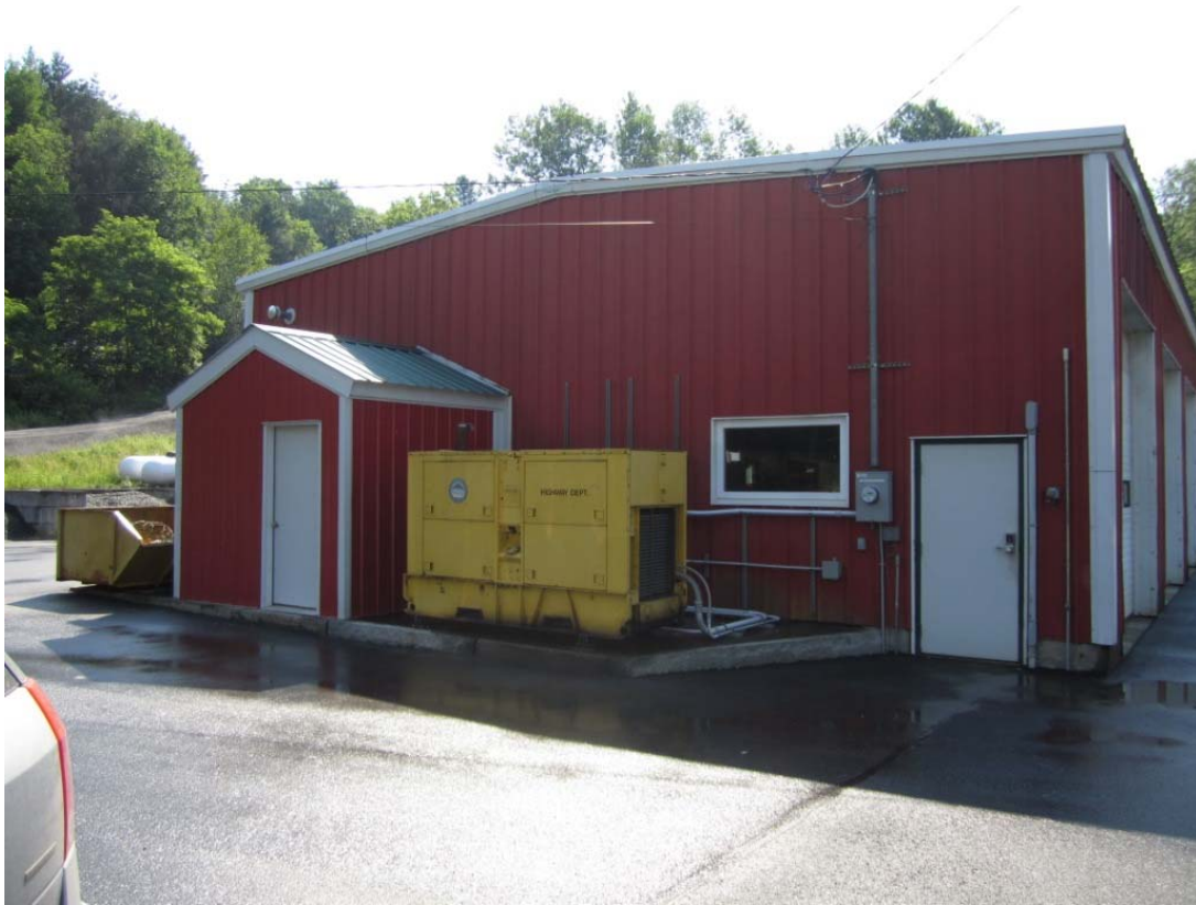
Photograph No. 19: Exterior of the existing building with solar panels.
